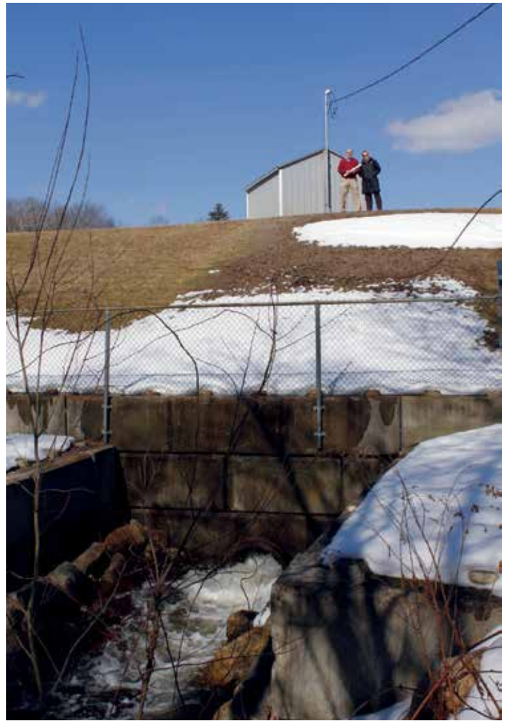
Figure 2. Gatehouse and sluiceway. Photo: Larry Cotton.
